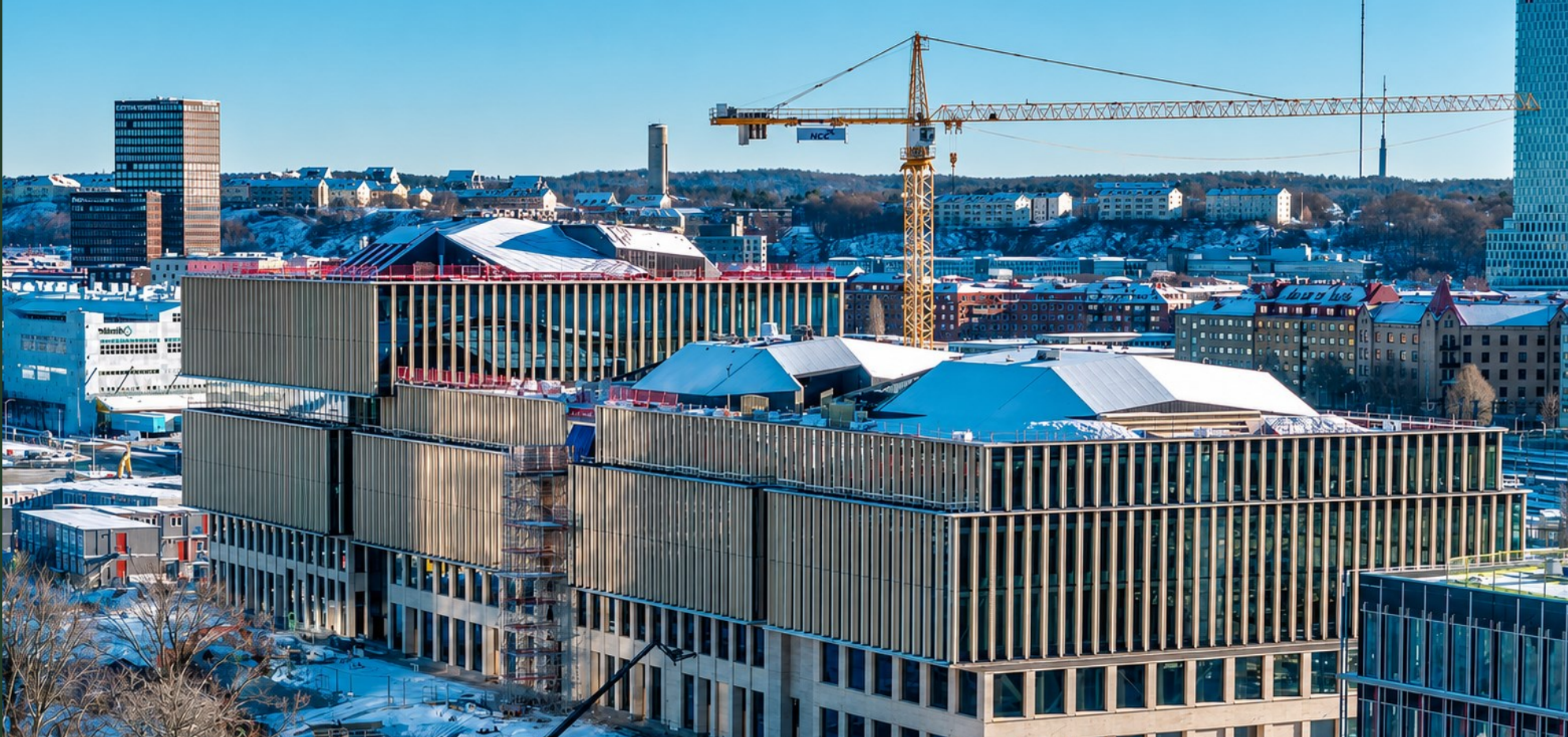
Accoya glulam facade material for the Park Central retail and office building in Gothenburg.
