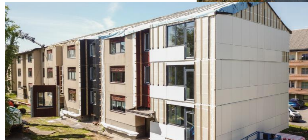
Renovation process 2021 summer
