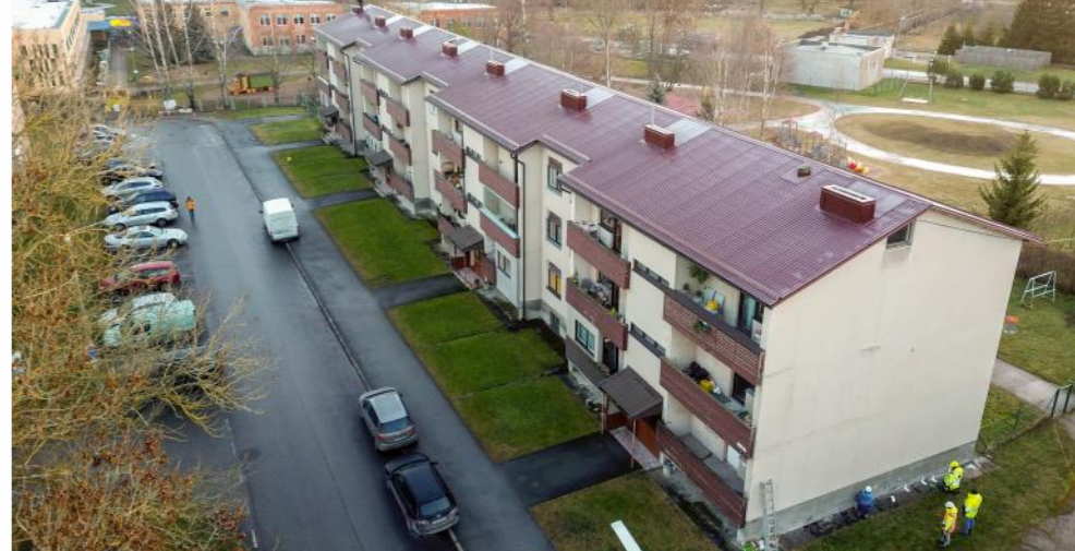
Apartment building before renovation 2021 spring
